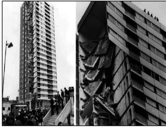
Figure. 2. Collapse due to column failure
