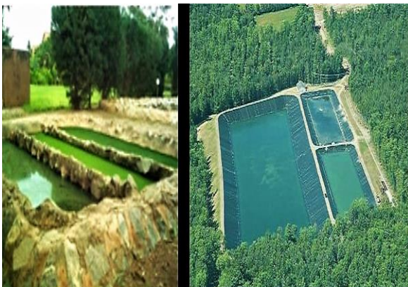
[Fig.05 Stabilization Pond]
