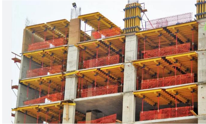
Tunnel formwork system
