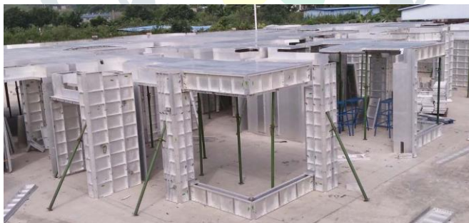
Aluminum formwork system
