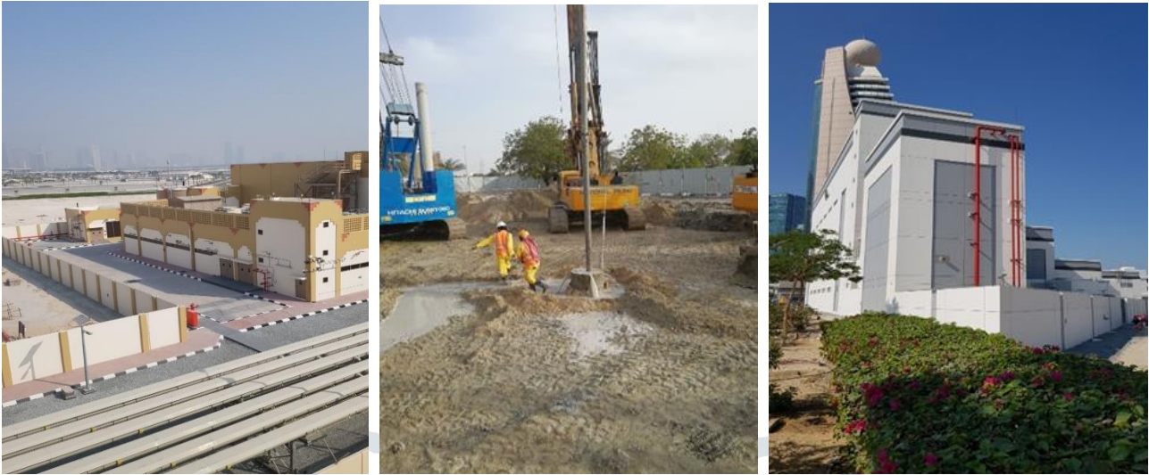
Construction of DEWA substations 400/132kV & 132/11kV substations in Dubai.
