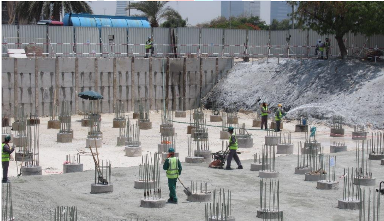
Building foundation processing details for RSHDPORT 132/11kV substation in Dubai.
