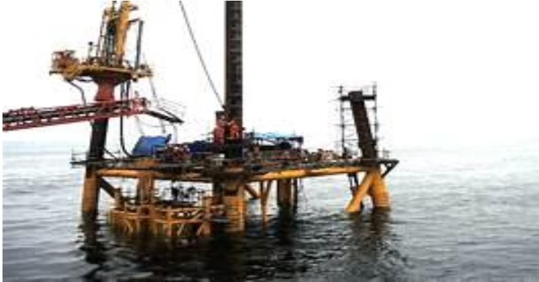
**FIG3.1: OFFSHORE STRUCTURE PILE DRIVEN METHOD**
