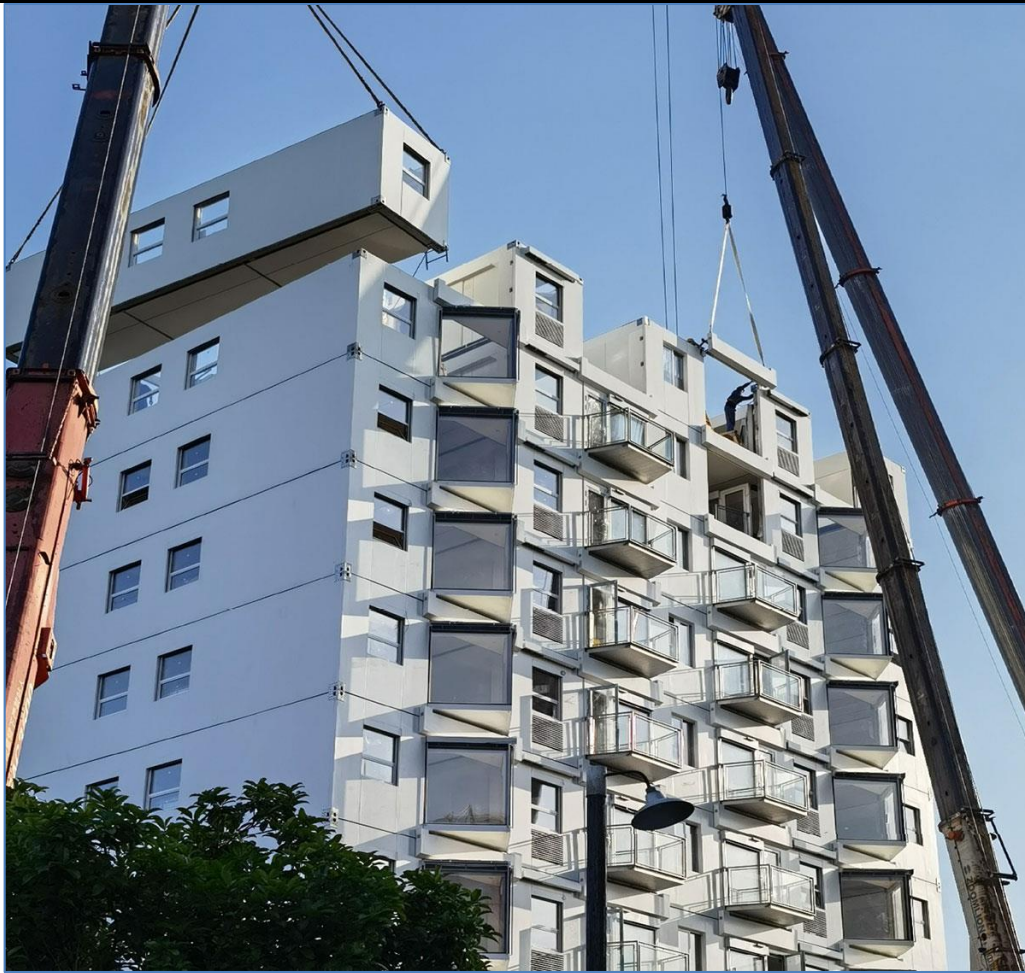
Figure 1: On-site construction of Living Building
