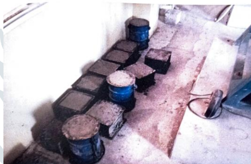
FIG 6: CASTING OF CUBES
