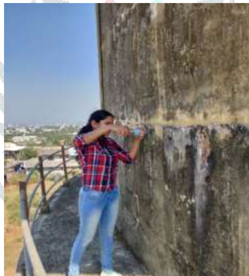
Figure 2 Performing rebound hammer test
