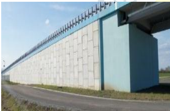
Fig. 1.1: Basic arrangement of reinforced soil wall with reinforcing element
