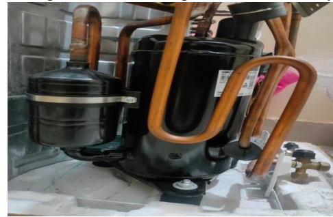
Fig. 2: R-32 Compressor
