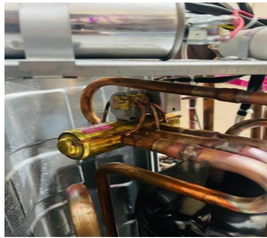
Fig. 5: Reversing valve
