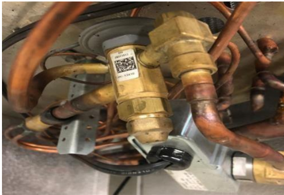
Fig. 4: Expansion Valve
