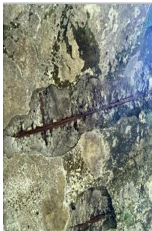
Fig.5. Spalled cover concrete and exposed reinforcement
