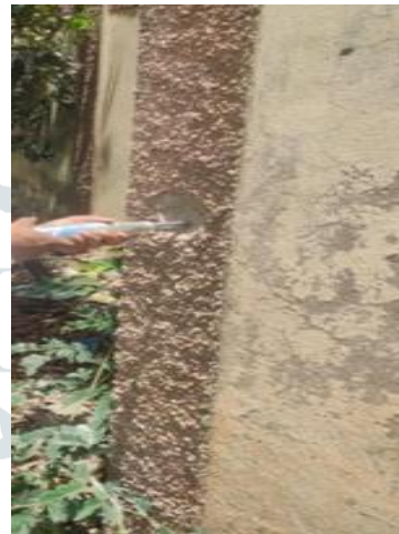
Fig.8. Rebound hammer testing
