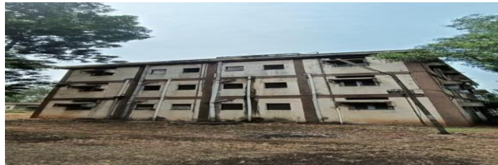
Fig.1. Existing Building: Case Study
