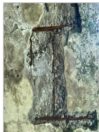
Fig.5. Spalled cover concrete and exposed reinforcement
