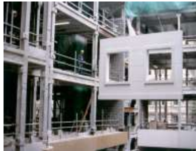
Pre-cast concrete infill panels
