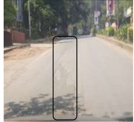
Fig. 3.2 At Ch 0+400 Up
