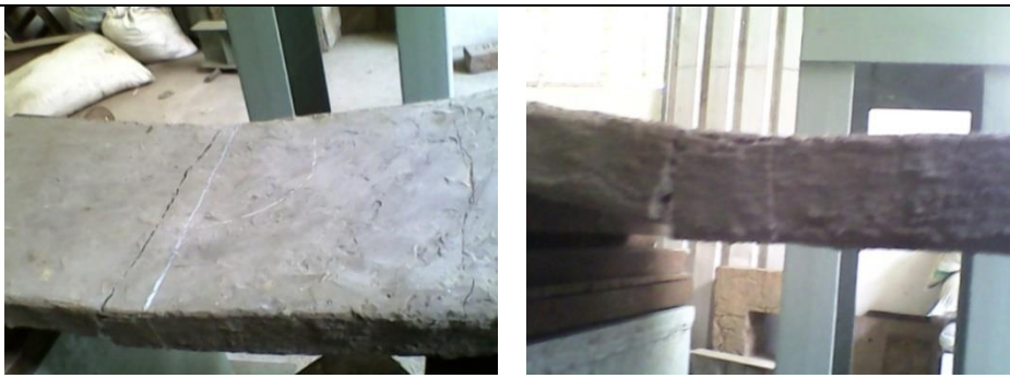
Slab Starts to crack at 0.6 KN, Initial Crack:0.6KN, Ultimate load:1.4KN
