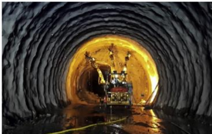
Figure 1: Tunnel construction site [11]
