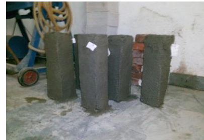
Fig 2.5 Column after plastering with cement mortar
