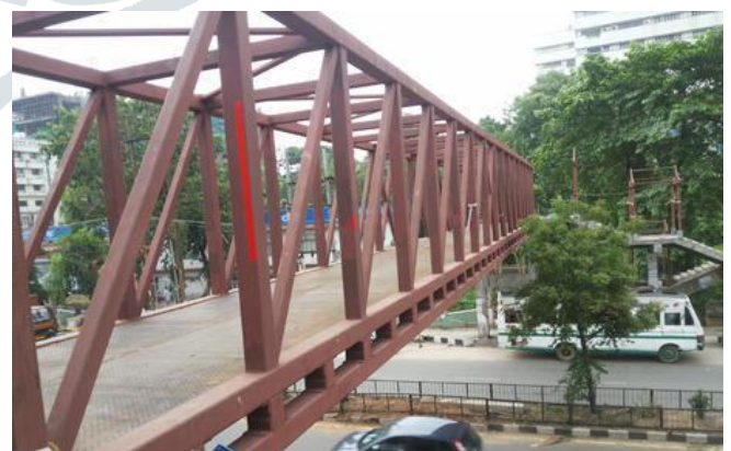
Fig. No. 1. Lattice Type Truss Pedestrian Bridge.
