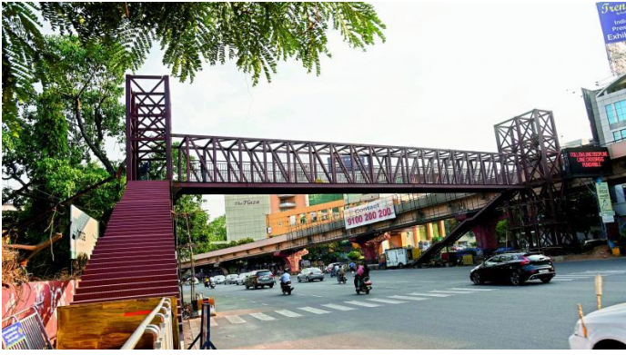
Fig. No. 2. Pedestrian Bridge
