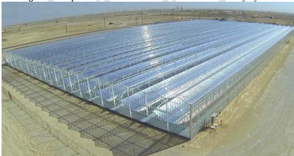
Fig. 5: Solar Power Production using Enclosed Trough.
