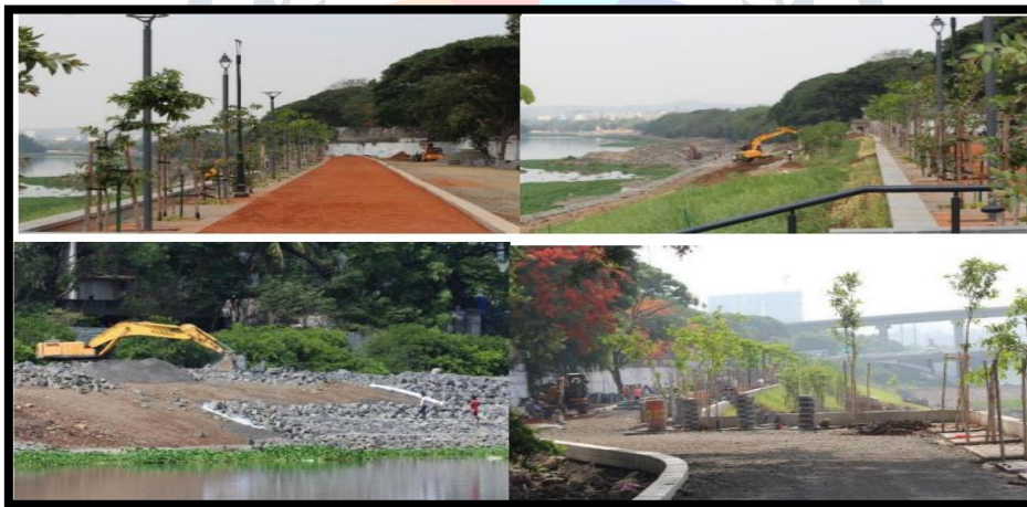
Fig : Sustainable river embankment
