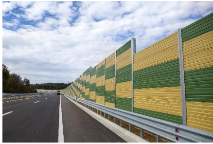
Fig 14: Non reinforced barriers
