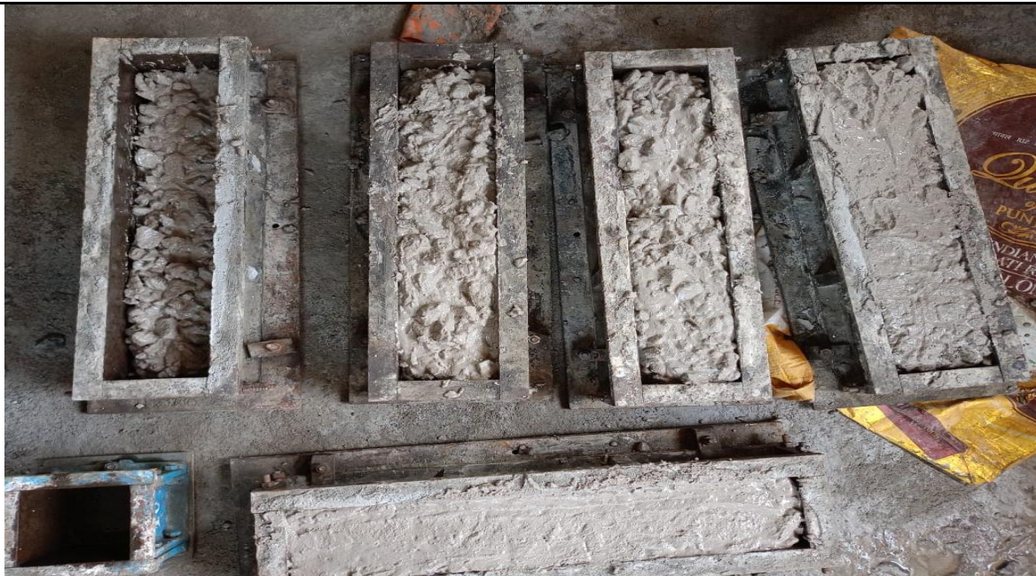
Fig.2 casting of beams
