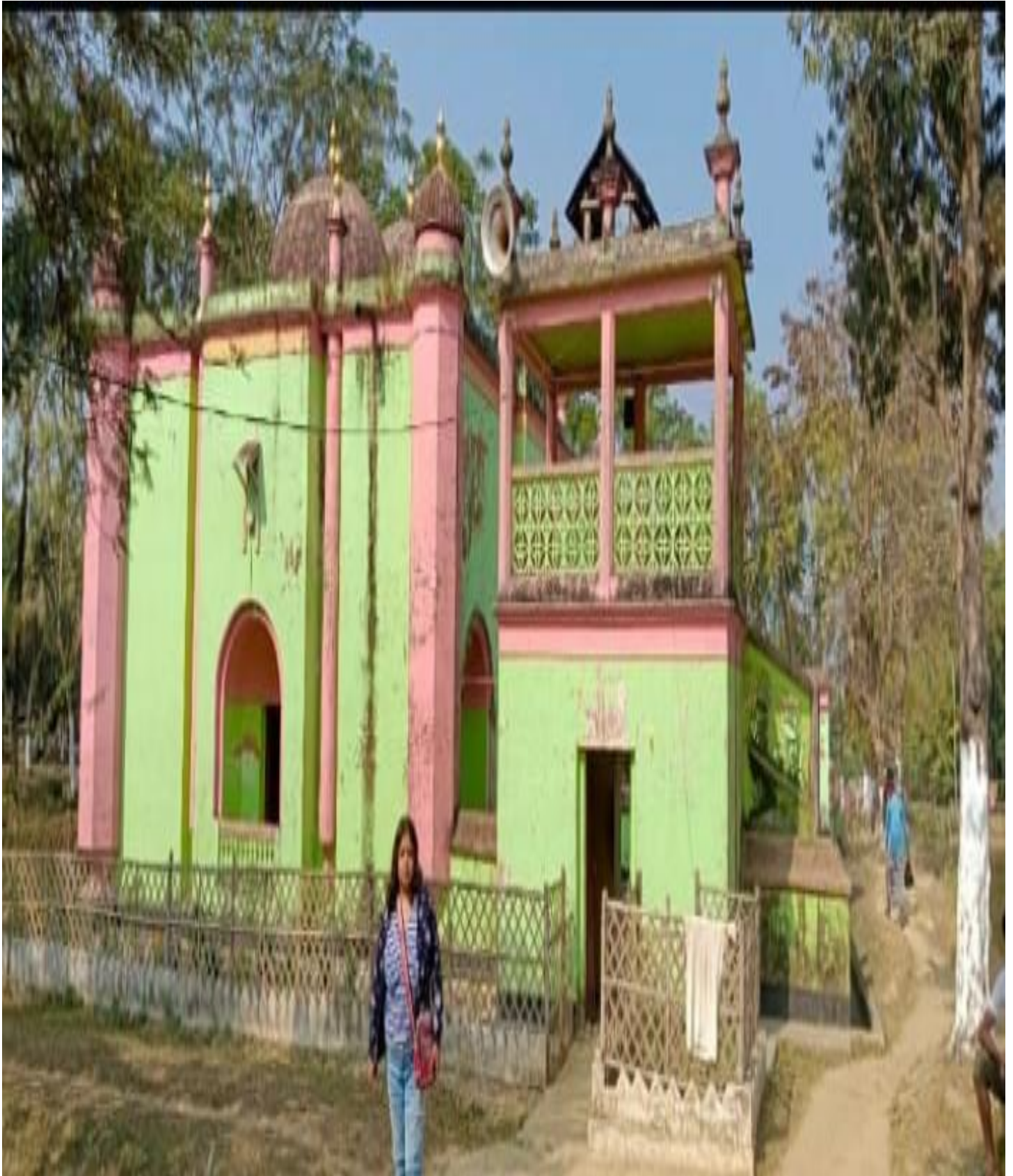
MOSQUE CONSTRUCTED BY GHULAM ZIRANI
