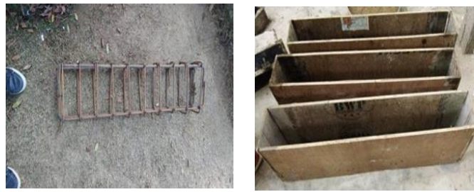
Fig 5 Casting of Beams
