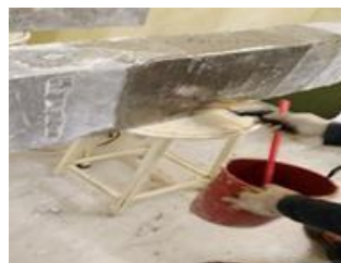
Application of Resin
