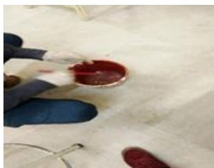
Mixing Epoxy Resin
