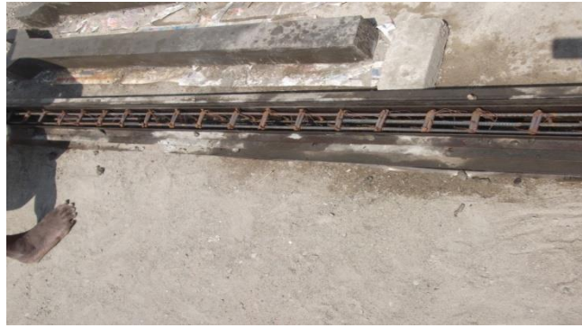
FIGURE 3.4 CASTING OF BEAMS
