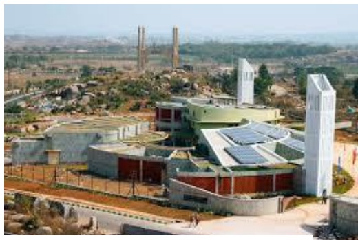
Figure 2, CII –Soharab JI Godrej green business center, Hyderabad, Source- Greenroofs.com
