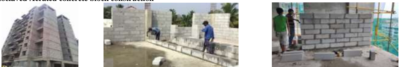
Figure 3: Construction in AAC Block
