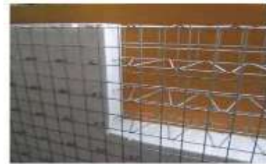
Reinforcing mesh expanded polystyrene core and diagonal wire
