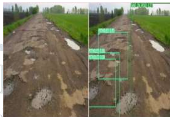
Fig.8.1 Road damages before and after detection
