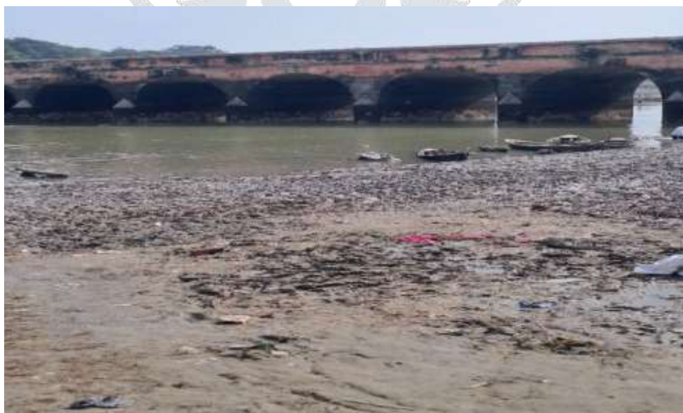
Fig 3: Image showing present condition of River Aami
