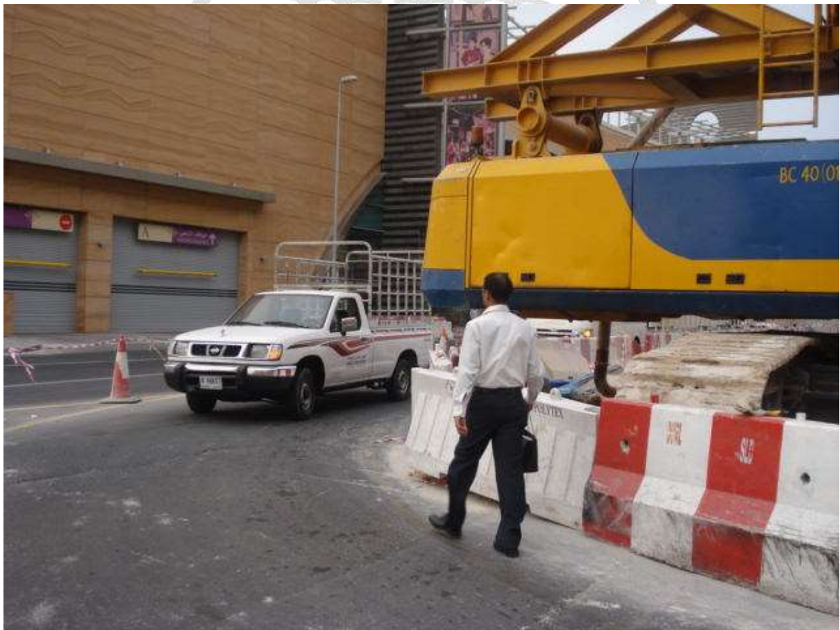
Crane operating near to public walkway and road
