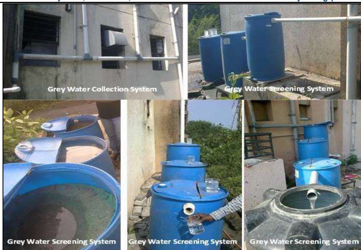
Fig. 1: Photos of grey water collection system
