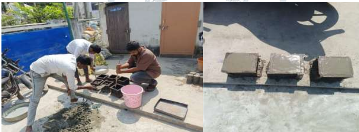
Fig 2 Casting of Concrete Cubes
