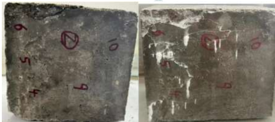
Fig-5 crack healing capacity of self healing bacterial concrete for day 1 and day 7
