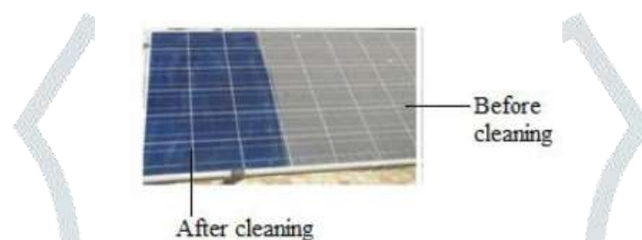
Fig.1. solar panel cleaning
