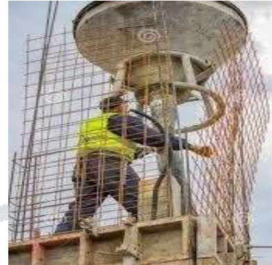
Fig 1c: Placing of Concrete
