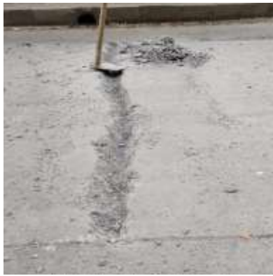
Fig 01: Making the groove
