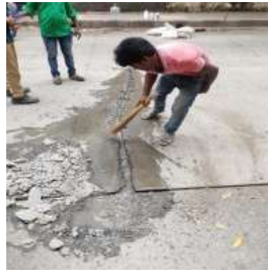
Fig 02: Cleaning the application surface
