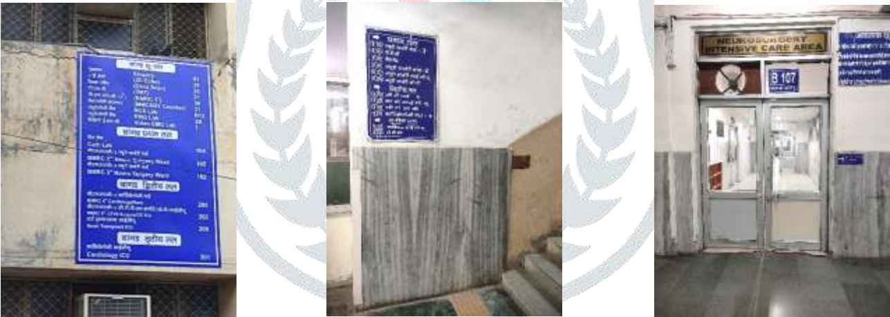
Figure 3: Different signage installation heights observed at SMS Hospital, Jaipur
