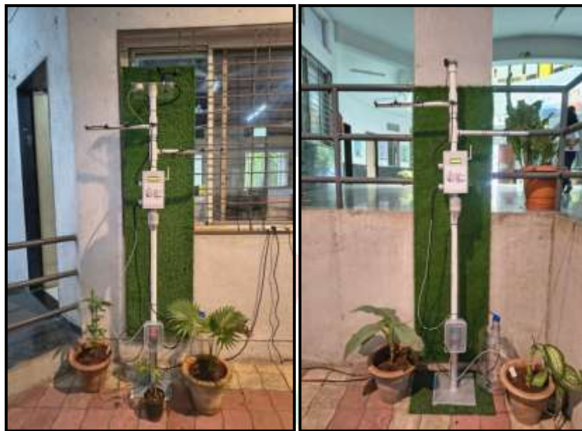
Figure 1: Master and slave node with installed sensor and control unit
