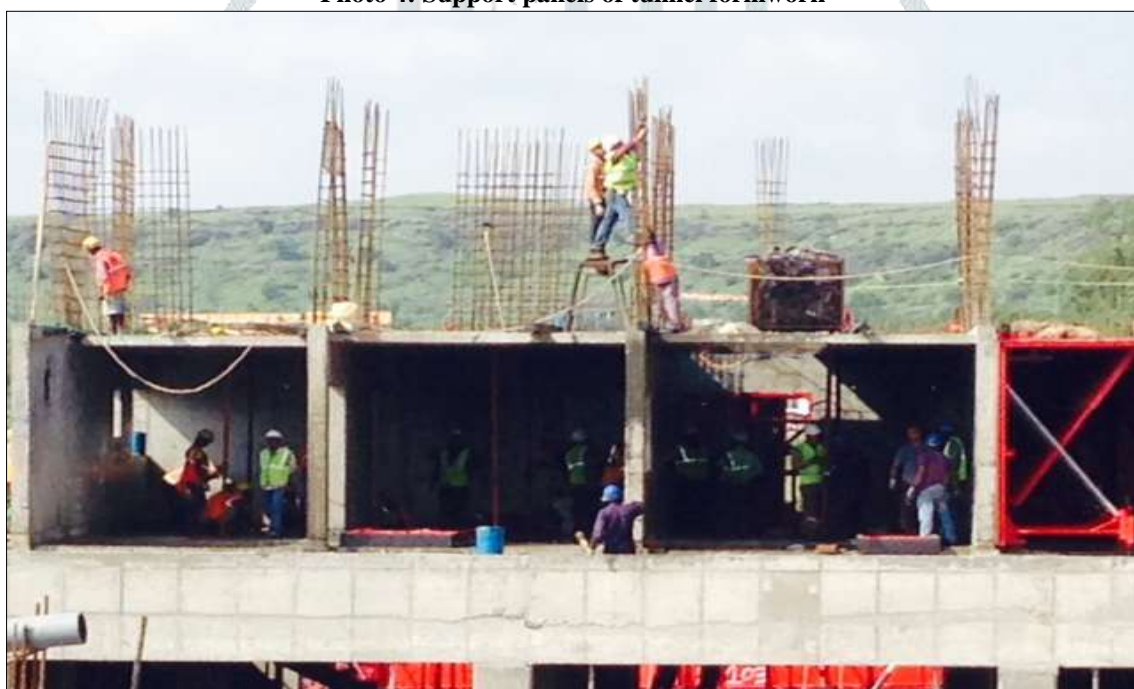
Photo 5: Slab after deshuttering formwork
