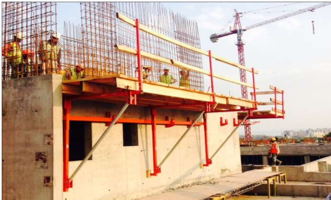
Photo 4: Support panels of tunnel formwork
