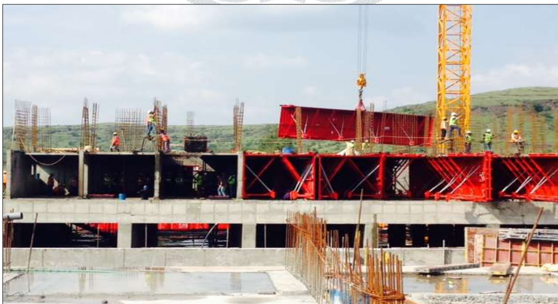
Photo 1: Erection of Tunnel formwork
