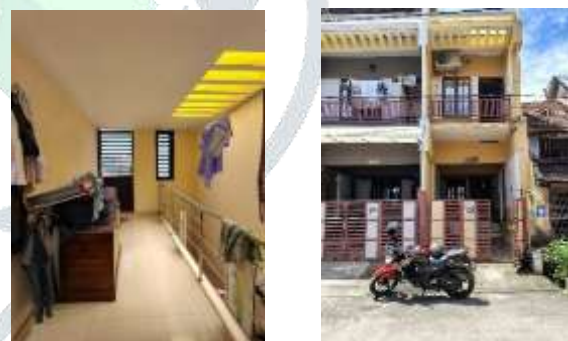
Fig.17 The internal skylight and external view of house no 6 (Photograph by author)
