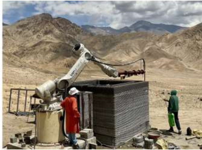
Figure 3 : Robotic arm manipulator constructing a defense bunker in Leh at 11,000ft, demonstrating 3DCP application in extreme climate [7].
