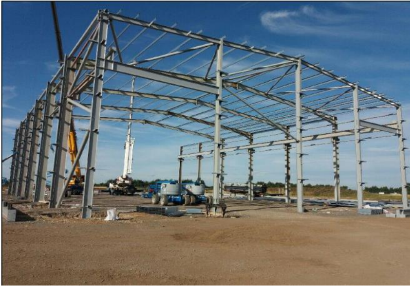
Figure 1: Erection of the NTS building primary structure 1
