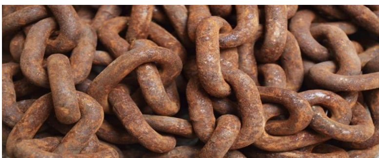
Figure (3): Uniform Corrosion
