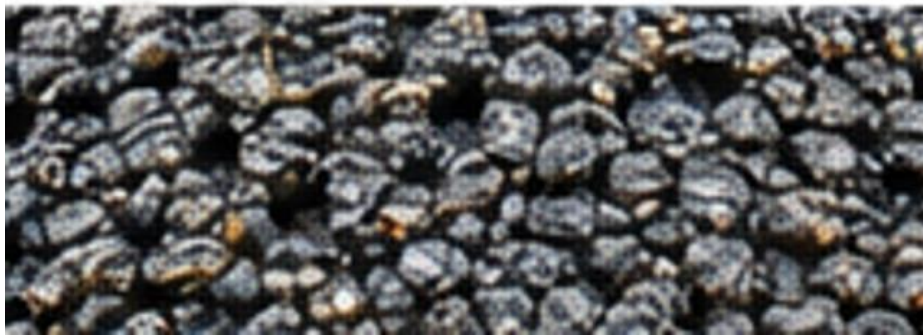
Porous asphalt surface (illustrative photograph).
