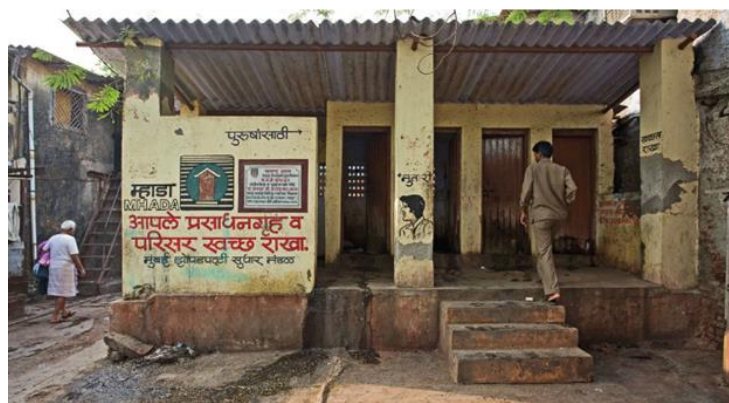
Figure 3: Community Toilet at Mumbai
