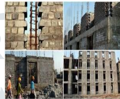
Fig.5.2.Construction of IIT Gandhinagar
