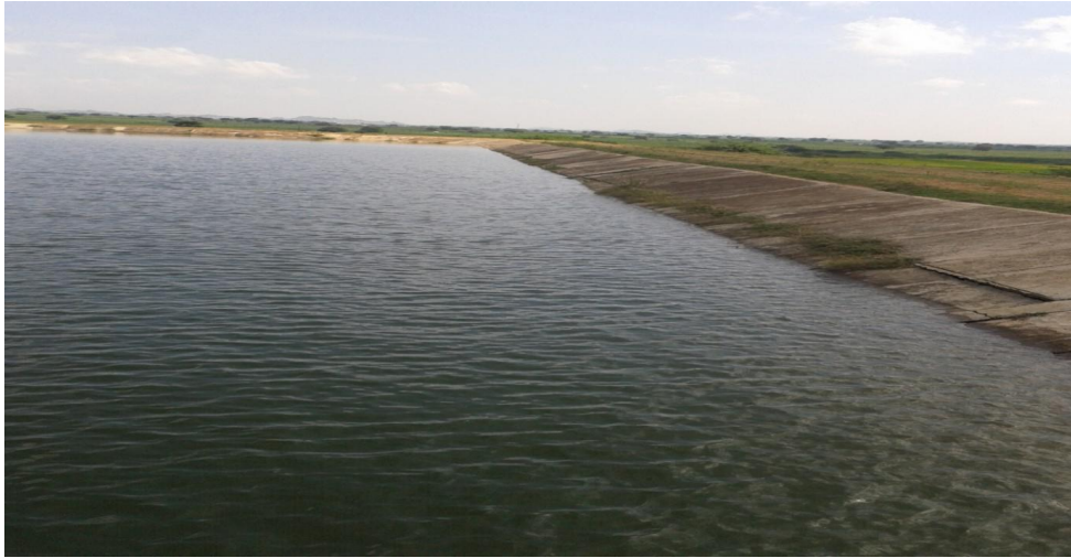
Figure 3.3.1 Upstream side of Embankment
