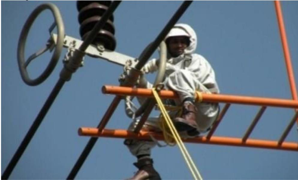
**Fig 1: Hot line inspection of transmission lines**
