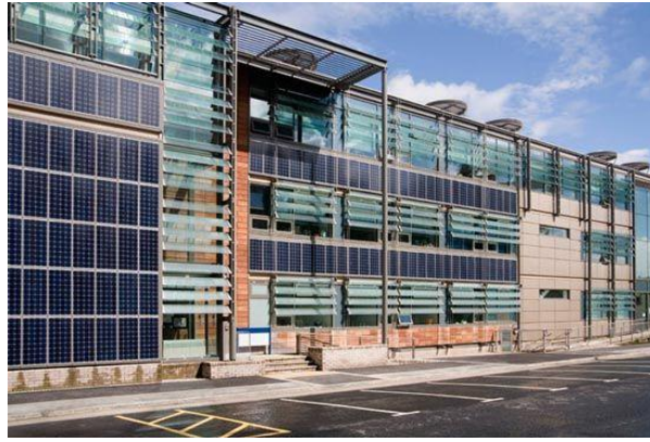
Figure 5. BIPV Cladding (Source: www.terrabeati.com )
