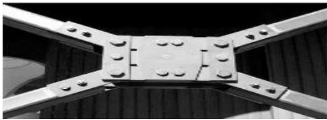
Figure-5: Friction damper
