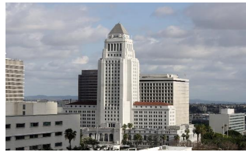
Figure-3: Building with base isolation
