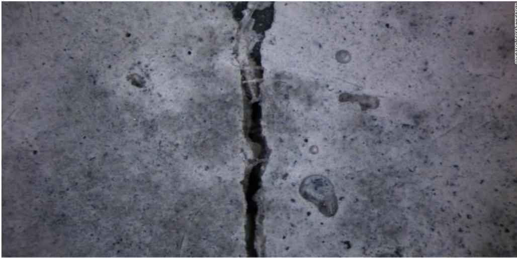
Figure: Crack develop in concrete
