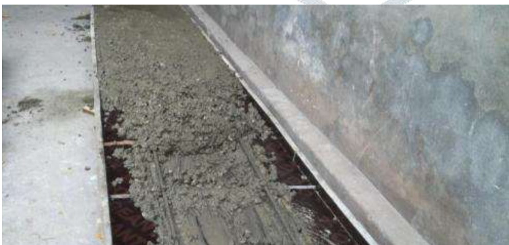
Figure 4: Concrete pouring in formwork for panel
